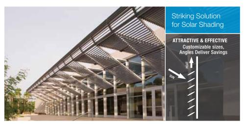
How: By shading the building façade, sun louvers control the amount of heat that can enter, helping limit cooling and heating loads. They can also ensure visual comfort by controlling glare. Sun louvers not only deliver outstanding functionality, but also create a distinctive look.
