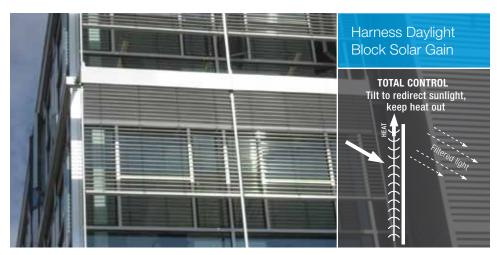
How: External motorized louvered blinds optimize performance by tilting to provide shading at varying sun angles. Similarly, daylighting blinds can tilt to bounce light off the ceiling and redirect it deeper into a space.
