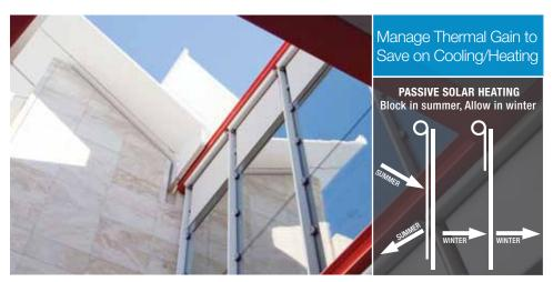
How: Motorized external roller shades manage the sun's energy very effectively, controlling light and heat before it reaches the building. With the proper shading fabrics, glare is filtered before it can impact learning performance and views to the outside are not interrupted.
